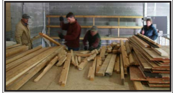
Pulling nails and cleaning up! (Iric, Russ, Harry and Shai)
